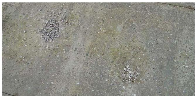
The surface of the concrete should be reasonably smooth and level with no noticeably high or low spots. Any loose or flaky areas of old adhesive should also be cleaned off.
