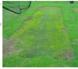
correct it by rolling from above. The cricket carpet would need to be removed and the base aggregate re-graded, levelled, and re-compacted before the cricket carpet is refitted.
