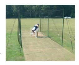
Here a ground socket is installed at each end of the net runs, with a steel post fitting into each socket. One has a basic strap winch attached; the other is an anchor post. A steel wire runs between the posts at high level, attached to the anchor post with a loop and to the strap winch with a clip, so the winch can tension the wire (a similar principal to tennis posts).
